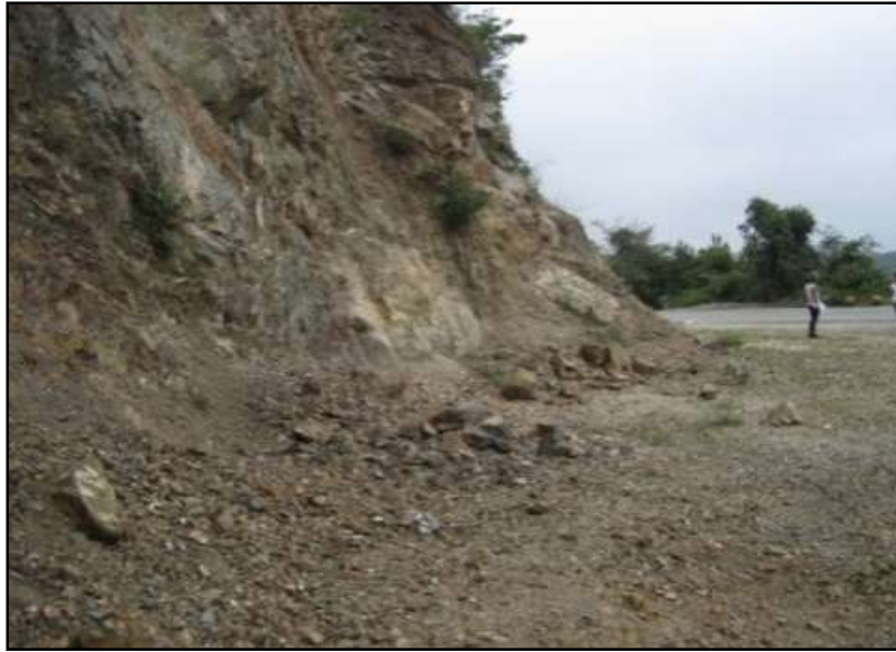
Figure 6 Rockfalls in the calc-phyllite unit at the western part of study area
