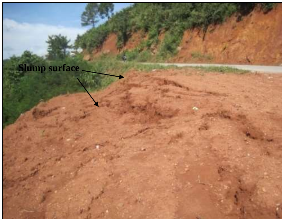
Figure 9 Occasional slump in residual soil at the eastern part of the research area
