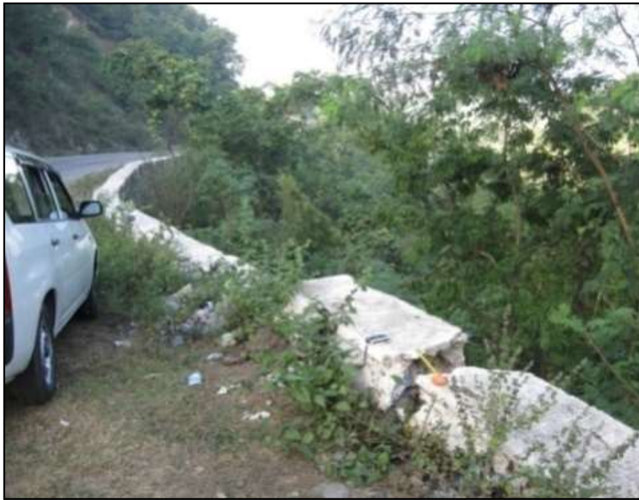
Figure 8 Creep due to stream bank erosion at the western part of the research area
