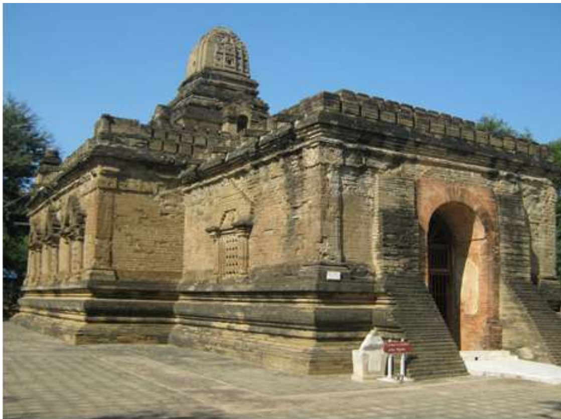
Figure1 Nanphaya, the Brahma's temple, south-east corner, sandstones backed by brick inside the temple, late 11 th Century CE or early 12 th Century CE, Bagan, Mandalay
