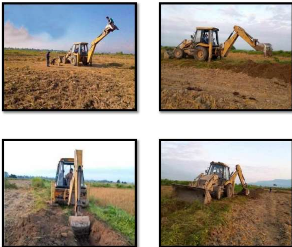
Figure 3. Re-excavation of Waste in the Farms and Paddy Fields
