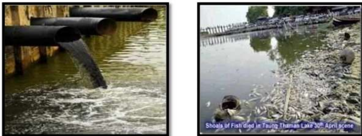
Figure 4. Wastewater discharge directly into water channel without pretreatment
