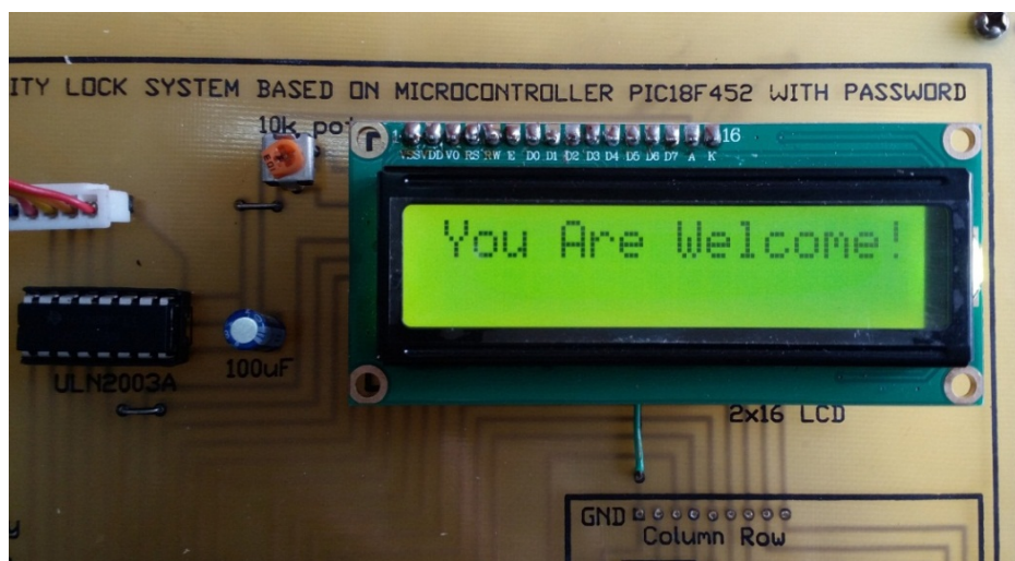
Figure 15 Initializing stage of security lock system
