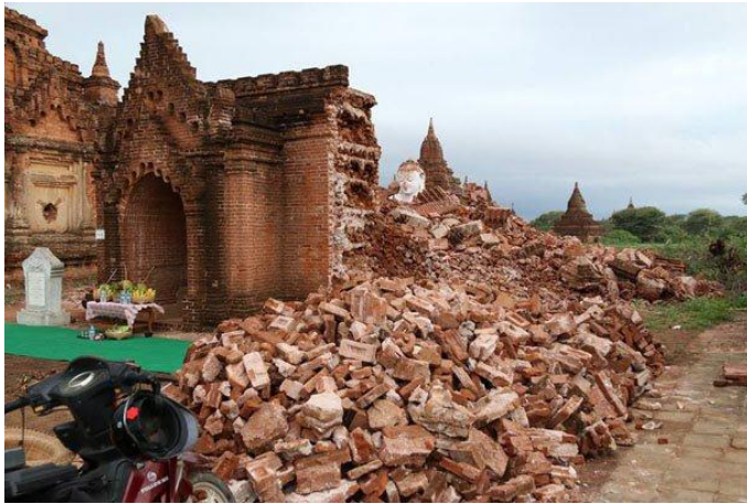
Figure 19: Subsidence in Temple No. 1752 at Bagan Area
