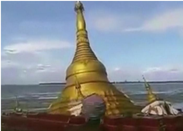
Figure 15: Subsidence due to Flash Flooding (Wash Landslide along the Ayeyarwaddy River Bank)
